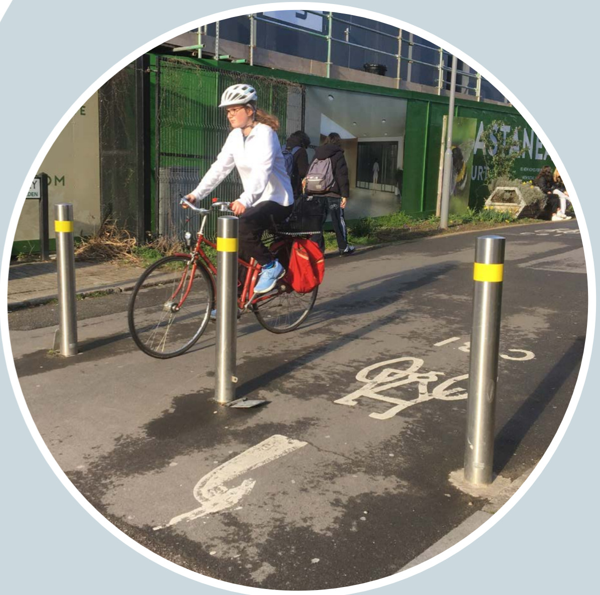
Fixed and lockable bollards, Cycleway 31, Kingston upon Thames
